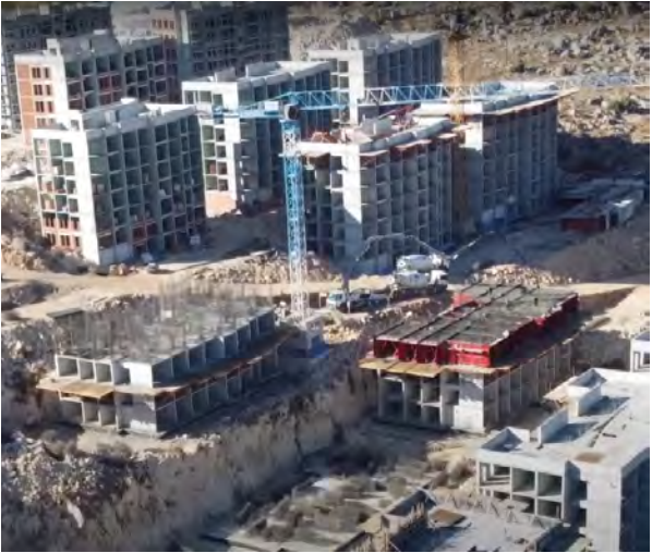
Earthquake Housing Const., Sept.'23
