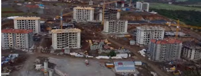
Earthquake Housing Const., July. '23
