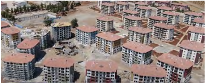
Earthquake Housing Const., Sept.'23
