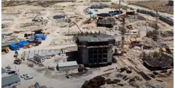
Earthquake Housing Const., June'23
