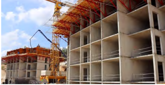
Earthquake Housing Const., June.'23
