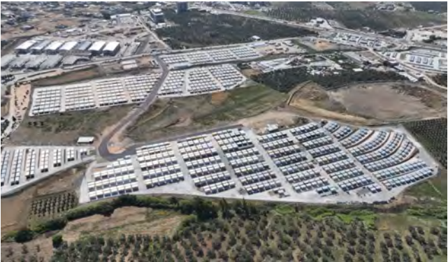
Hatay Qatar Funded Container City
